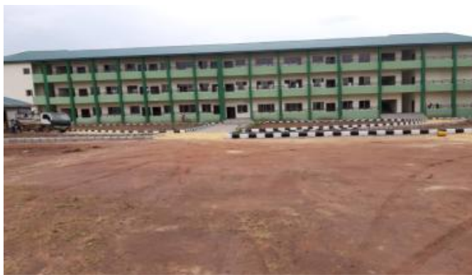
Newly-Built Classroom Block
