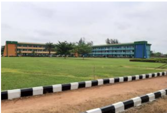
Some of the existing Crawford University classrooms
